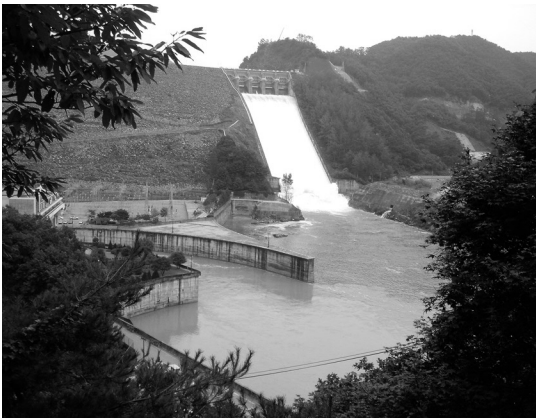
Fig. 4. The inflow of turbid water into Soyang river (전, 2007).
